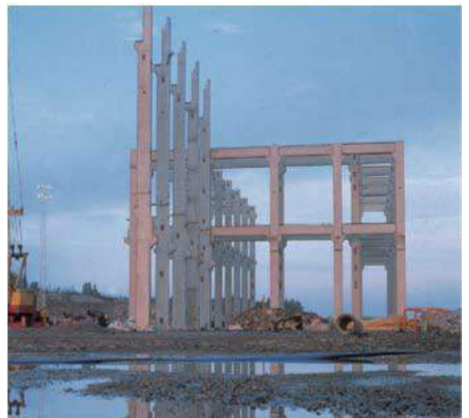
Precast columns during erection.
