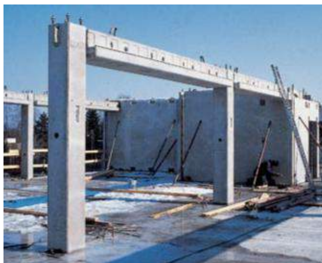
Building with central core and hidden beam-column connections.
