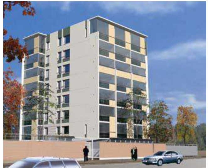
Load-bearing cross-wall system with hollow-core floors spanning over 10 to 12 m.
